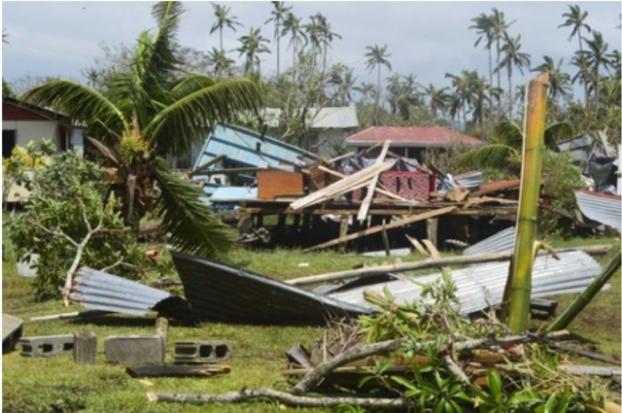
Figure 2.2 Debris close to the shore in Fiji after Hurricane Winston.
